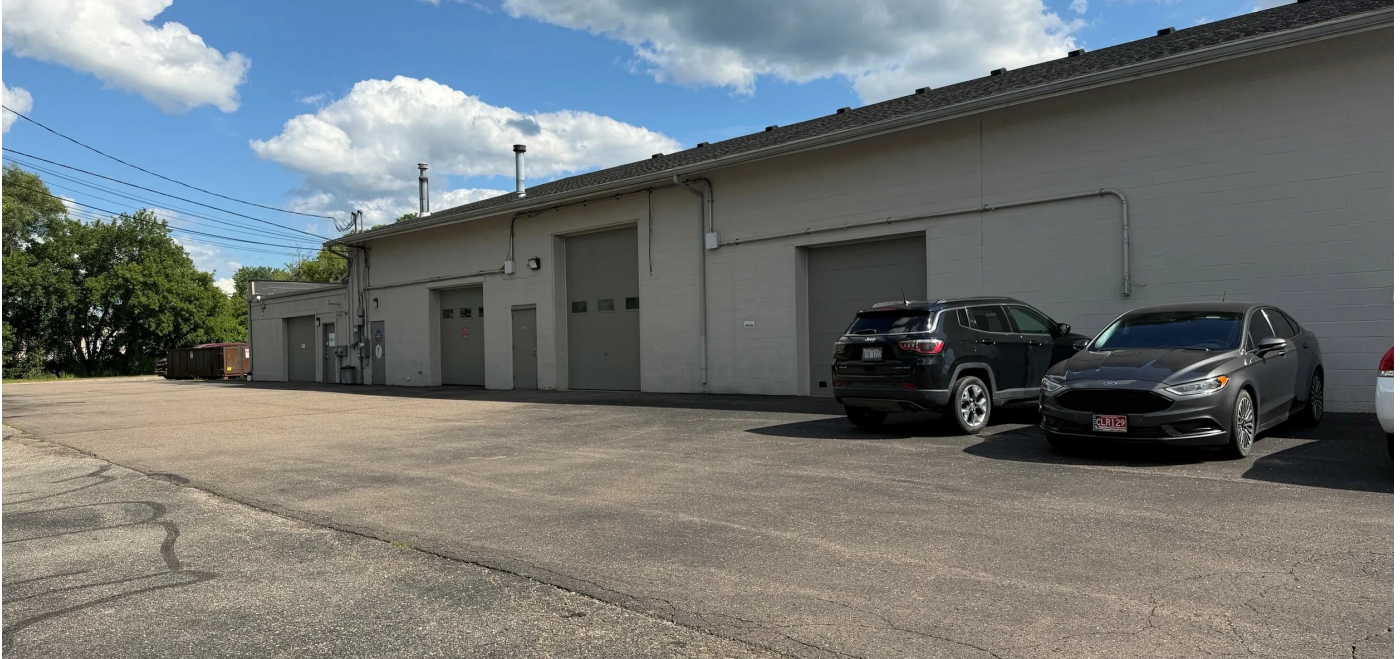
BUILDING #2 - Rear Building Photo
