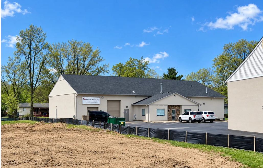
BUILDING #1 - 9897 Weber Street (Back Building) - 9,180 SF
